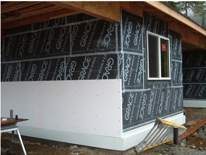
A house using the REMOTE wall system building technique under construction in Juneau, Alaska.
