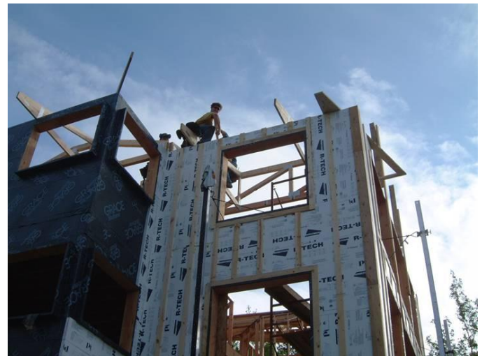
REMOTE wall under construction in Fairbanks, Alaska showing vapor barrier, insulation, window framing and furring in place for siding.
