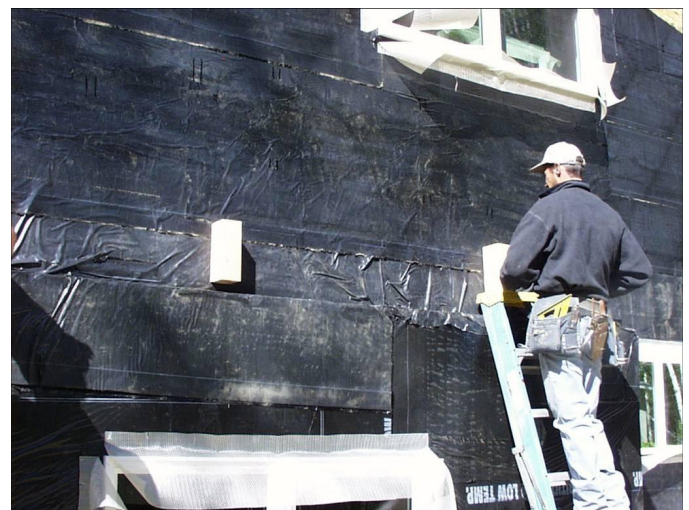
REMOTE wall under construction showing exterior vapor barrier, deck blocking & window detail.
